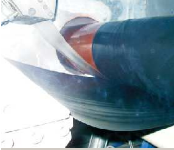
Three Layer Polyethylene (3LPE)
