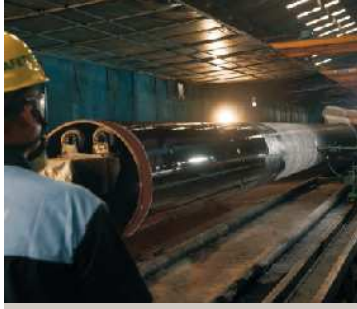
External Epoxy Coating
